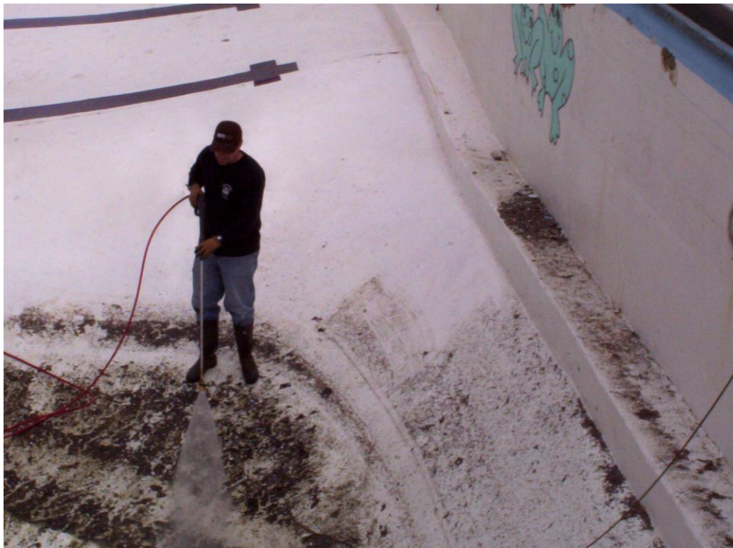
Ted Dean power washing the pool and getting it ready for some new paint.
